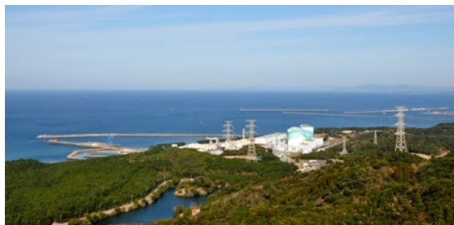
The two-unit Sendai plant
