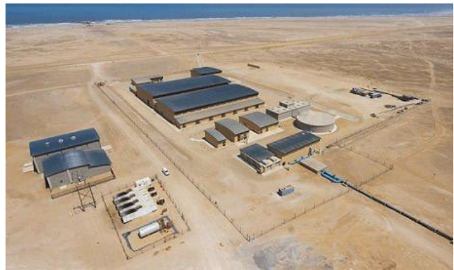
AREVA's water desalination plant in Namibia
