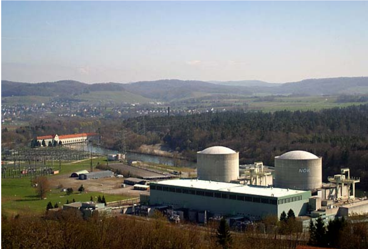
Beznau nuclear power plant
